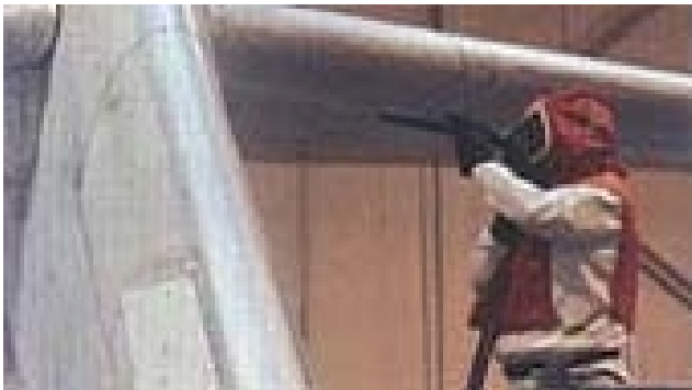
Dry Media Blasting Process
