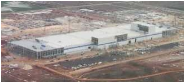
Fig. 1 Aerial view of factory under construction
