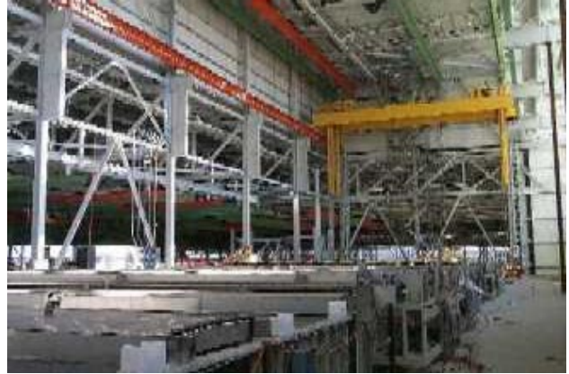
Fig. 2 Mezzanine view of chemical processing line.
