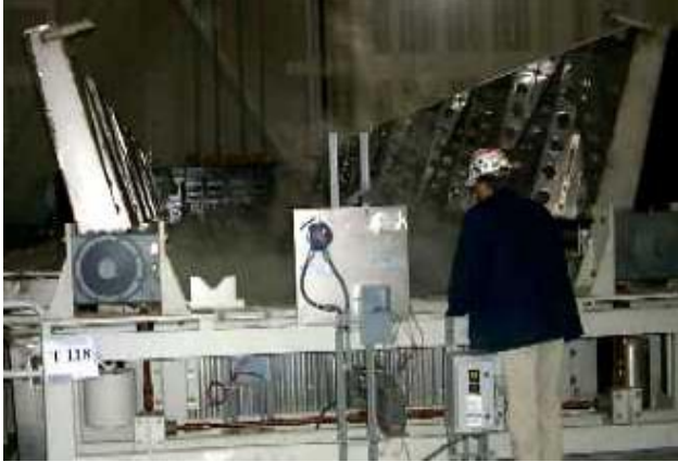
Fig. 4 Mezzanine view of typical tank lids
